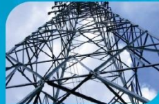
Latis Towers (Power & Telecommunication)
