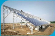
Solar Structures & Other Steel Fabrication Work
